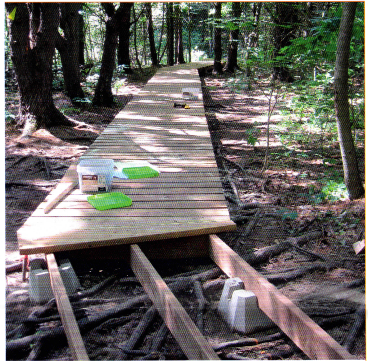
Boardwalk over exposed roots, part of trail improvements
