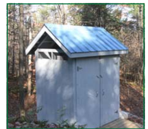
New Comfort Station
